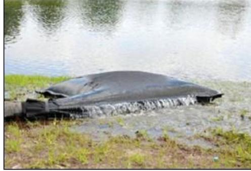
Plate 4-7 Silt bag under inspection
