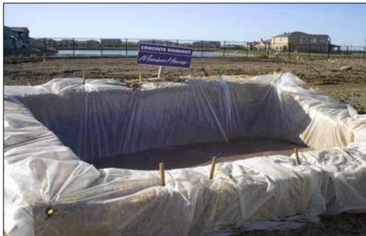
Plate 4-3 Concrete washout area
