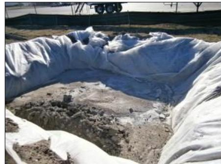
Plate 4-4 Concrete washout area
